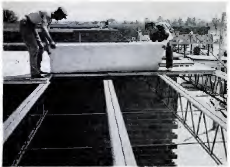
Left, torch has little effect on fireproof roofing material. Right, covering roof with wood-fiber planks
